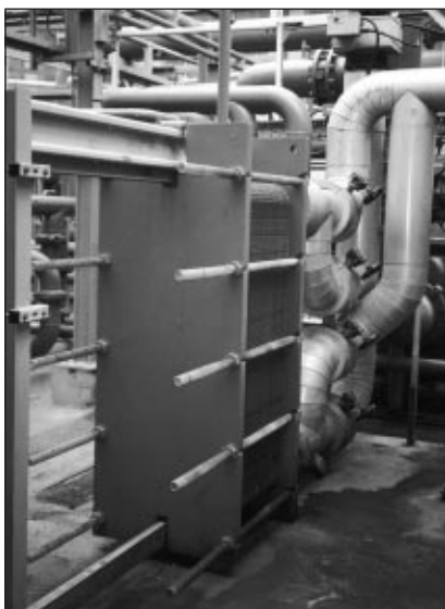
Figure 10 Plate heat exchanger
