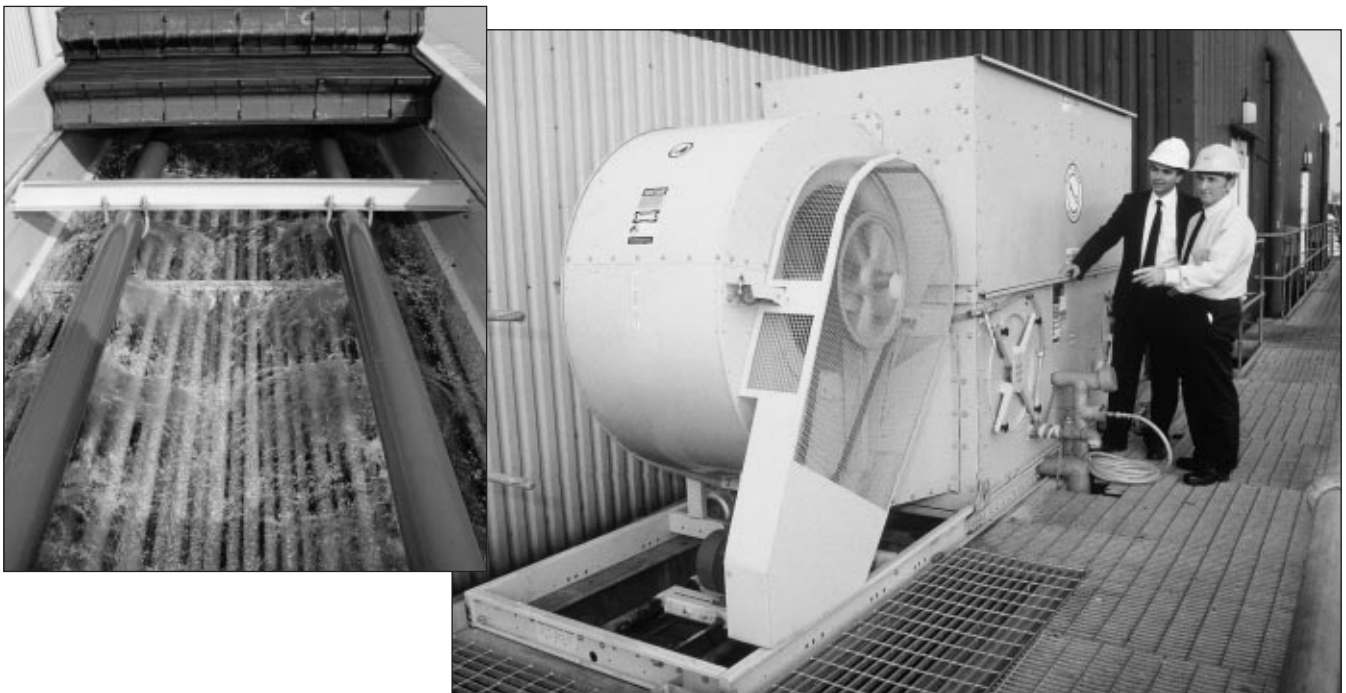
Figure 25 Evaporative condenser
