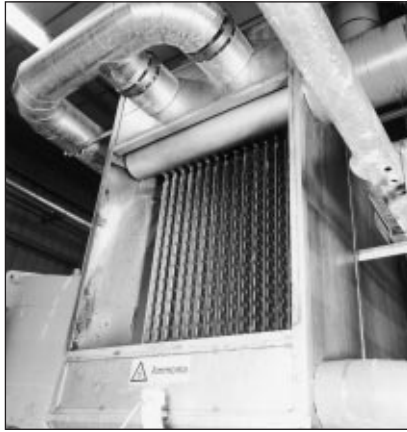
Figure 11 Baudelot cooler
